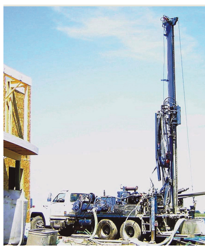
Ener-West residential geothermal system installation
